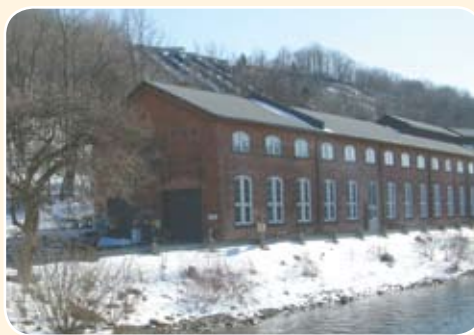
Decew Falls original building. IEEE Hamilton Section
